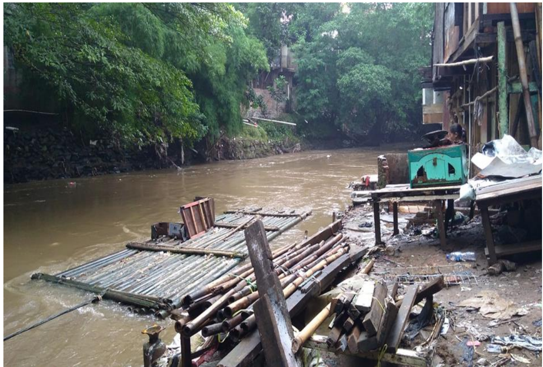
Figure 1. A raft with toilet destroyed by flood
