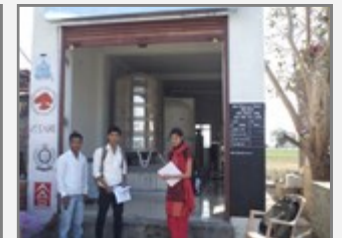
Amrut RO Plant
