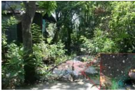
Polluted water sewages with bad smell and breeding sites for mosquitoes in section 3
